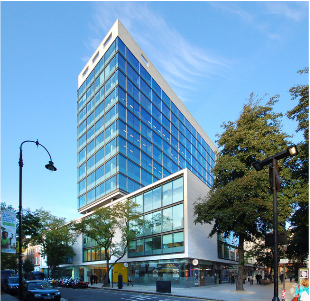
The Met Building
